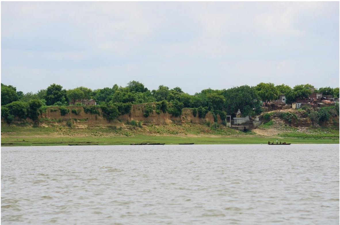
Image 76 : Eroded Bank Near Tanda Kalan [Right Bank]
