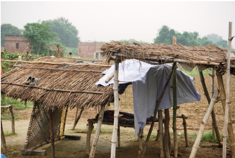
Image 58 : Temporary Shelter with Thatched Roof of Dried Saccharum munja Note : Pucca Houses in the Background on the Island
